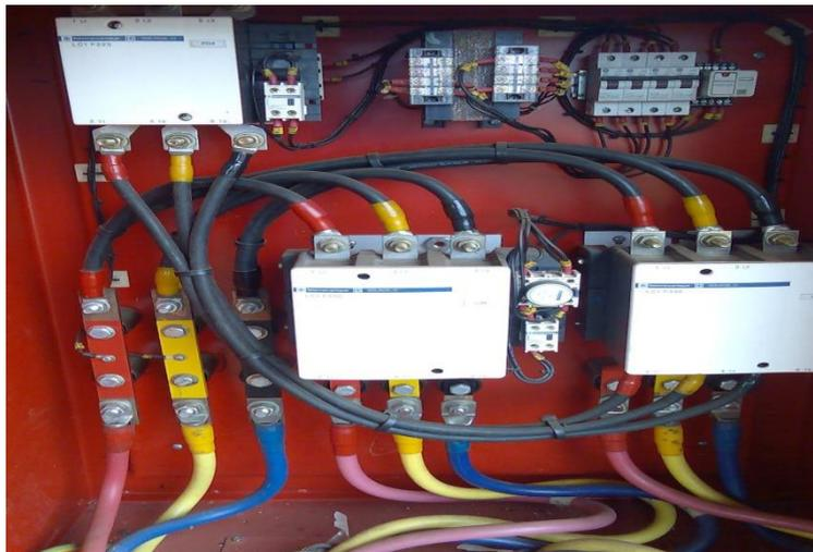
*Gambar Star Delta Electric Fire Pump*
